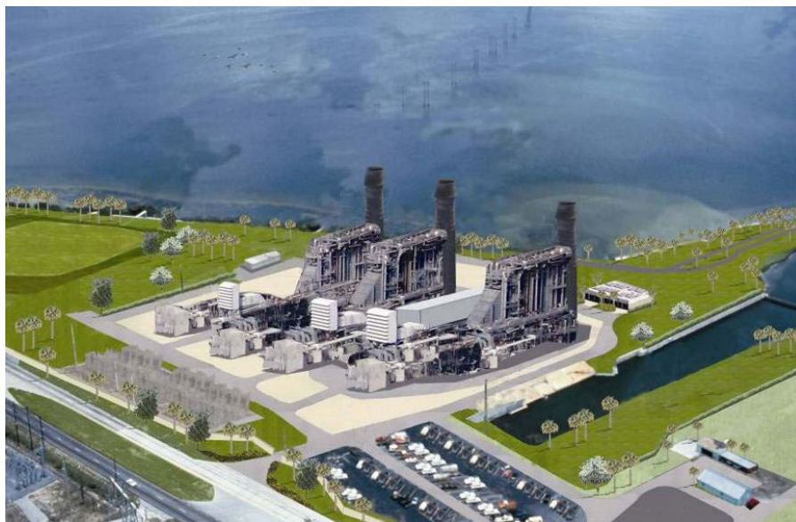
FPL's Cape Canaveral Next Generation Clean Energy Center, 2013
